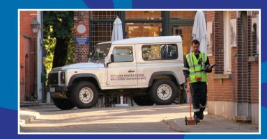
Leak detection on underground pipelines
